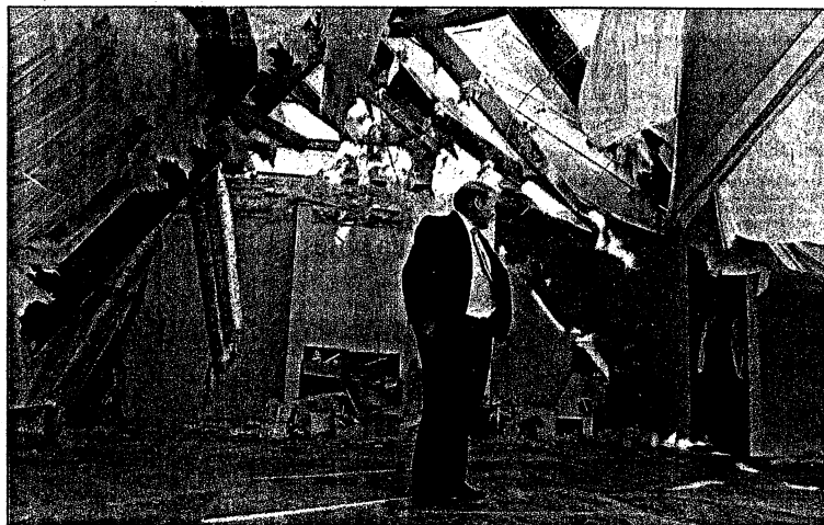
The Rev. Anthony Pemberton and his wife, Michelle, of the New Life Apostolic Church survey the tornado-damaged second floor of the church. On Nov. 10, the Mossy Grove, Tenn., church was near the center of the hardest-hit area of the tornado but did not fall. "It was like the Lord wrapped his arms around us," said parishioner Jody Summers.
